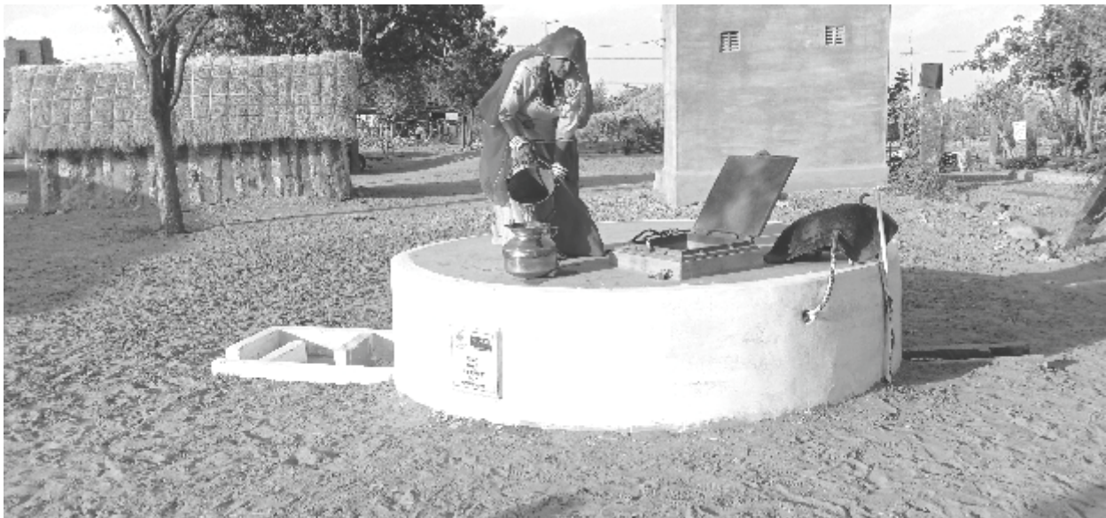
A newly constructed taanka in Andasar village, Baap block, Jodhpur district
